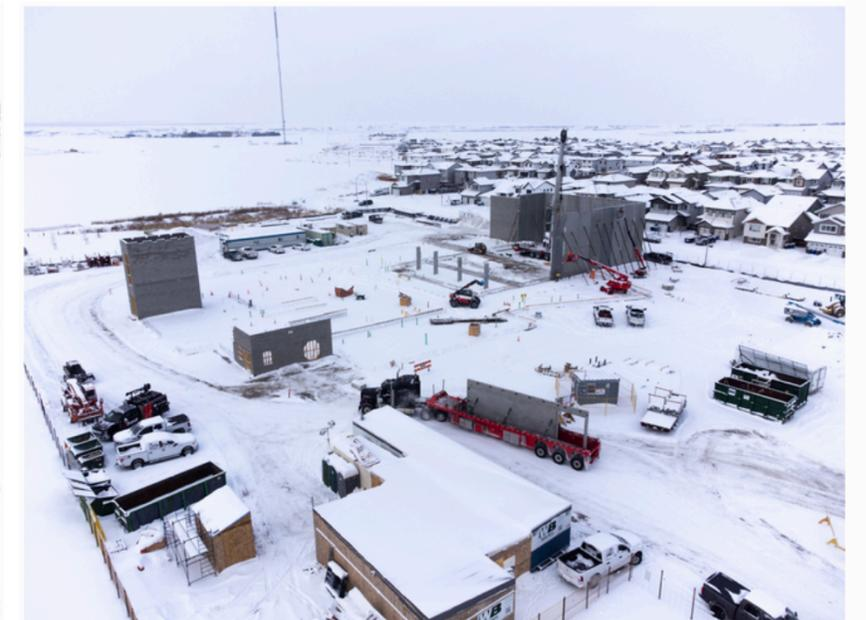
Concrete load-bearing walls are tilted to avoid winter construction slowdown
