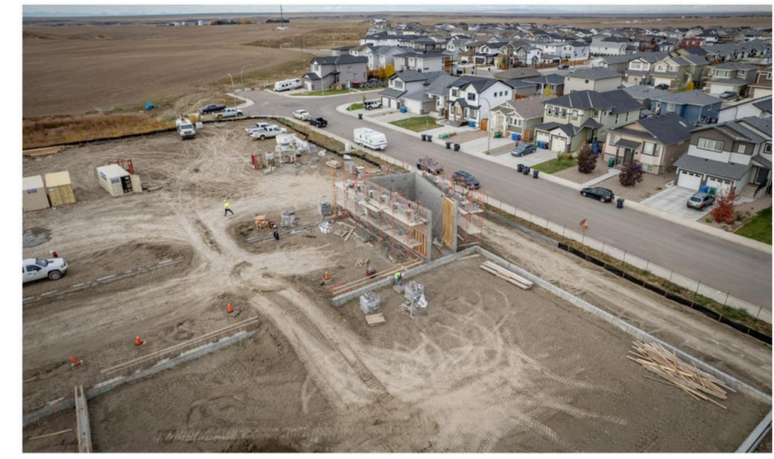
Foundations are completed and the concrete blocks stairwells are prepared
