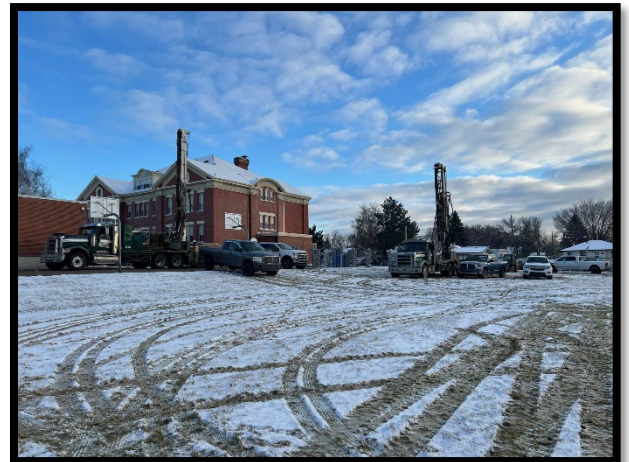
Geotechnical testing for Galbraith Modernization
