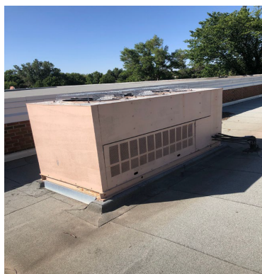
Fleetwood Bawden Condensing Unit Replacement before and after
