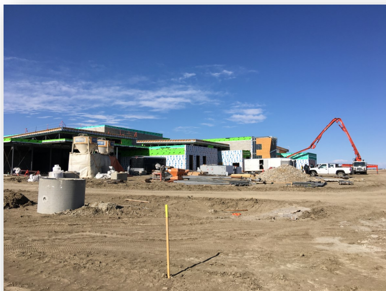
Senator Joyce Fairbairn Middle School in construction 2016 The school opened September 2018
